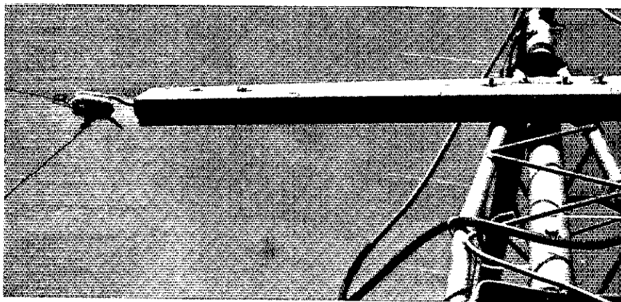
Fig. 2 — Detail of how the antenna is mounted to the top of the tower. TV-mast clamps are used to secure the wooden insulator.
